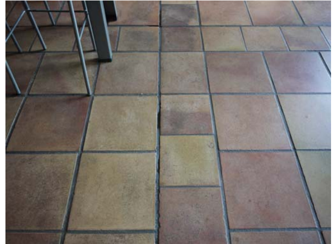
Foyer/Bar, Detail Bodentrennfuge
